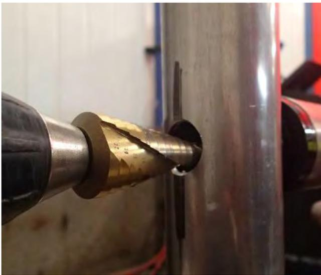
26. Use a Stepped Drill Bit to drill the  $\text{\O}4\text{mm}$  pilot hole out to  $\text{\O}24\text{mm}$ .
