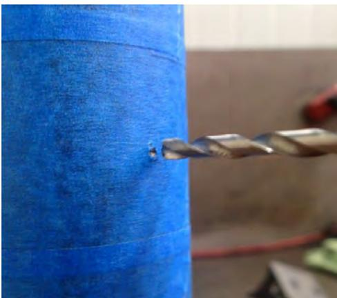
31. At the location of the Centre Punch mark, use an Ø4mm (or similarly sized) Drill Bit to drill a pilot hole through the front face of the Bull Bar outer frame.
